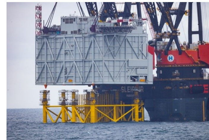
August 2024 installation of an HVDC offshore converter platform at RWE's Sofia Wind Farm, off the coast of the United Kingdom. (Image credit: RWE)
