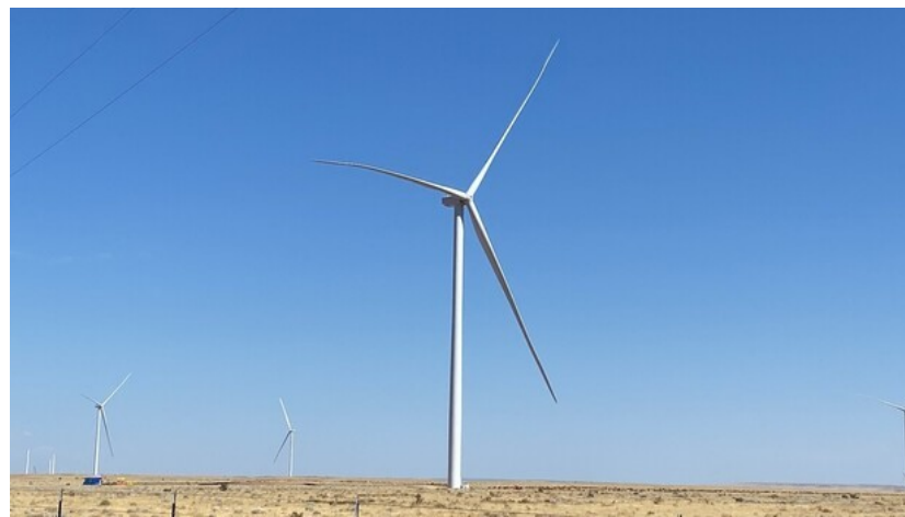
First of 674 3.6MW-154m workhorse turbines that will provide 2.4 GW+ of power installed at Pattern Energy's SunZia Wind Project in New Mexico, expected to be the largest wind project in the Western Hemisphere.
