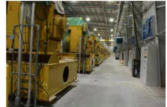
Construction of our 175 MW Yellowstone County Generating Station
