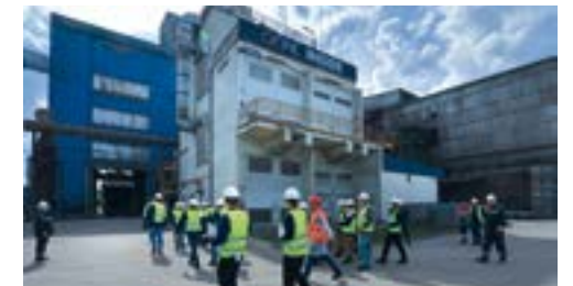
ABS Sisak / Croatia Hybrid by design, the Q-One power feeder ensures the most efficient digital control of the EAF, with a negligible impact on the power grid.
