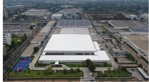
Targeting 100% renewable electricity by the end of this fiscal year through the largest scale installation of solar panels within the Sony Group
