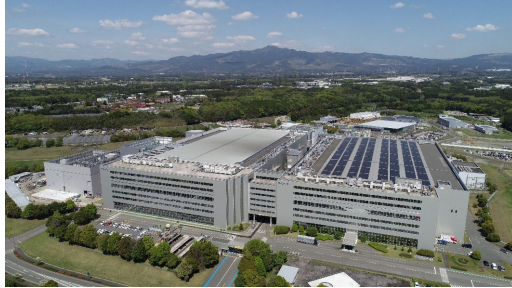
Expansion of solar panel installation
