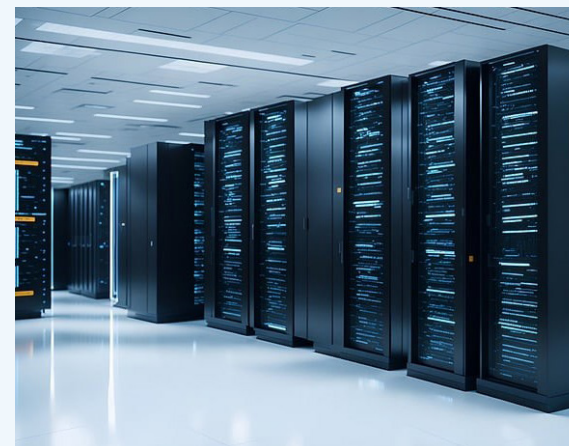
There is increasing demand for air conditioners at data centers
