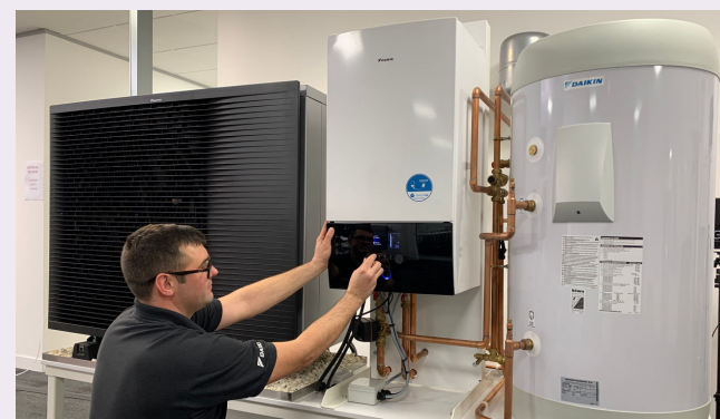
Training on installation and maintenance of heat pump space and water heaters
