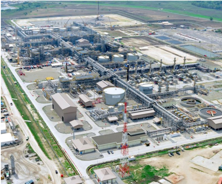
Banyu Urip Central Processing Facility, Indonesia
