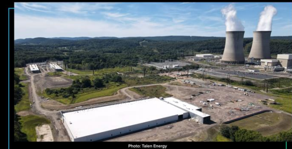
Photo: Talen Energy
