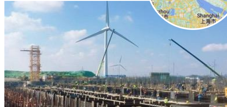
Site Construction Progress
