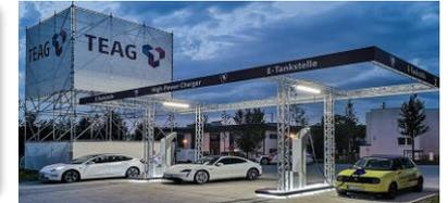
“ “Microgrid” pilot project in Berlin where ads-tec Energy’s HPC charging solution is used. The **technological heart of the system are the two ultra-fast charging points**, which are supplied by a buffer battery. With this... we can also provide ultra-fast charging in places where the local power grid does not provide the technical or commercial prerequisites”
