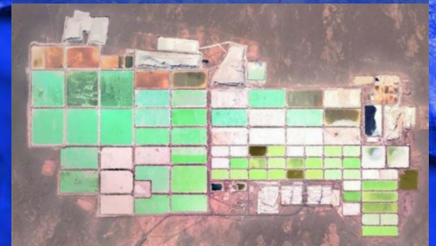
Multiple Evaporation Operations
