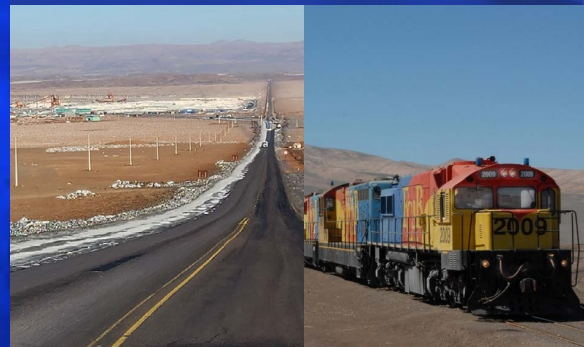
Quality Road & Rail Infrastructure
