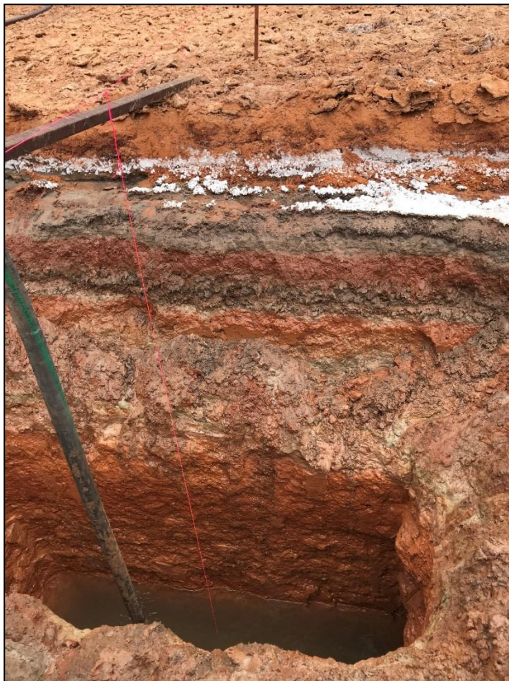
Figure 3: Test pumping of a test pit excavation
