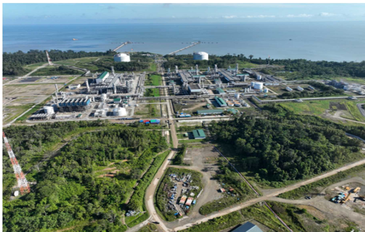
A bird's-eye view of the Tangguh LNG Terminal
