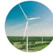
Each MW of Wind Power 120-180t steel
