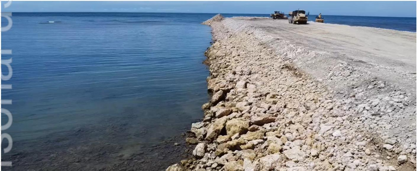
Above: Wharf completed to Stage 1 (rubble core)
