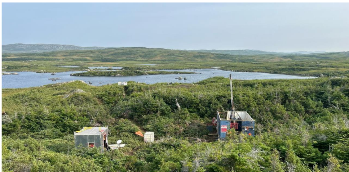
FIGURE 4: DIAMOND DRILLING AT O-2 WEST TARGET
