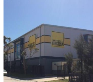
National Storage Kumell marked for further expansion and additional marine storage
