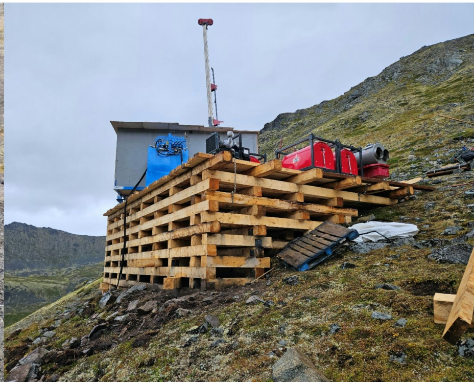
Drill on Deck and drilling away end of August 2023
