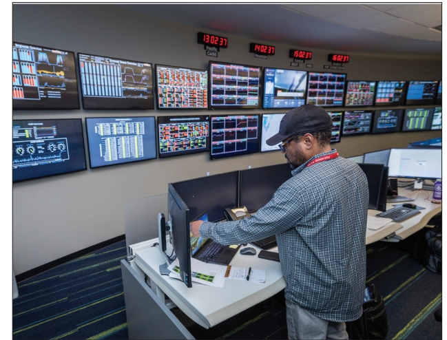
Through the integration of remote monitoring, modeling, and diagnostics, Vistra’s POC identifies, forecasts and advises plant personnel of emergent issues impacting production before more serious conditions happen.
