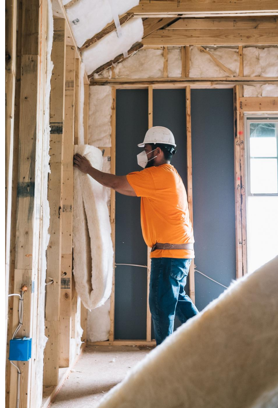
TruTeam residential insulation installation in progress.
