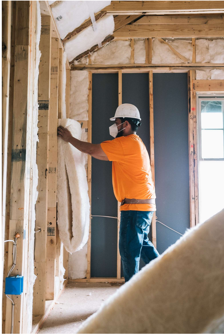
TruTeam residential insulation installation in progress.
