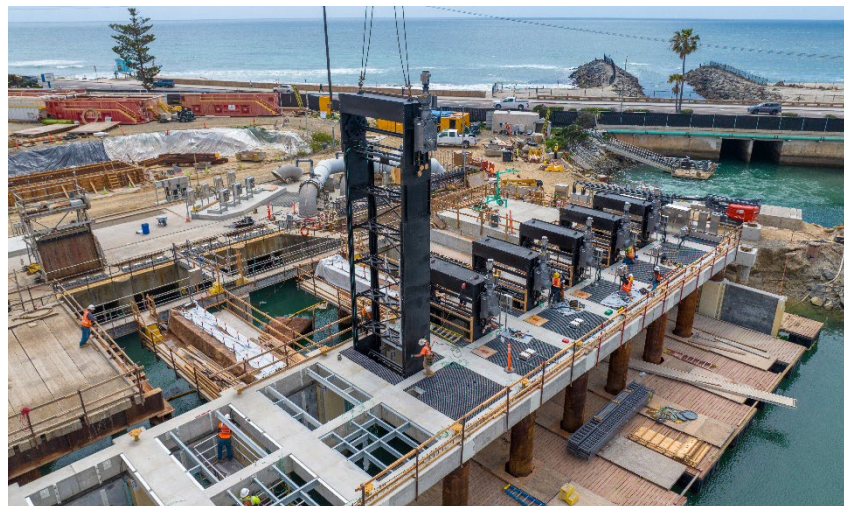
Claude "Bud" Lewis Carlsbad Desalination Plant intake construction.
