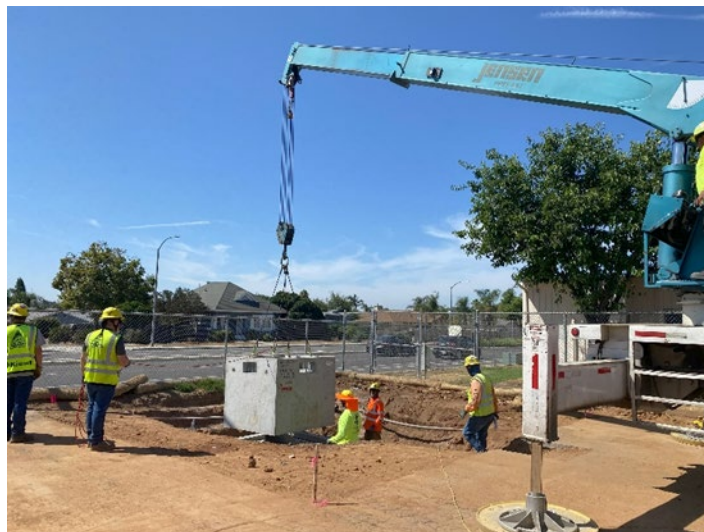
First Aqueduct Structures Rehabilitation Hubbard Hill South.
