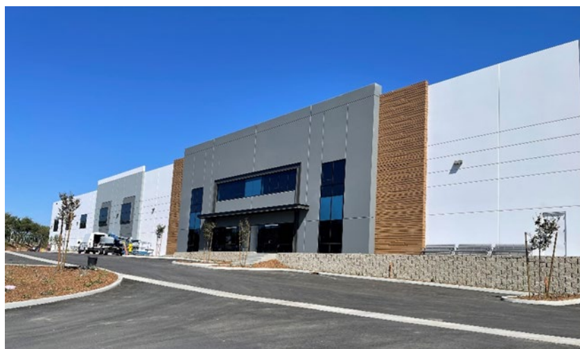
Operations and Maintenance Department Facility.
