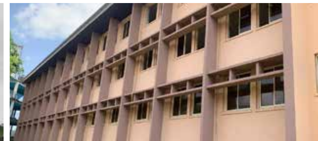
Obstetrics and Gynaecology Ward (Block C) of the Lagos University Teaching Hospital (LUTH) Commissioned: 27th March 2023
