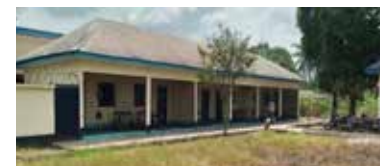
Ubeta CDF Project: Renovated Corpers Lodge
