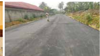
Rumuji CDF Project: 1Km Road
