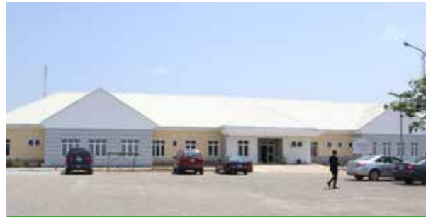
Maternity Centre at the University of Abuja Teaching Hospital (UATH) Commissioned: 18th November 2022
