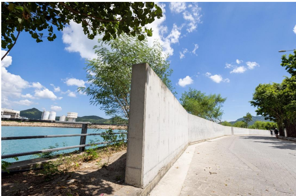
Flood walls of about two metres high have been erected at key locations in Lamma Power Station.
