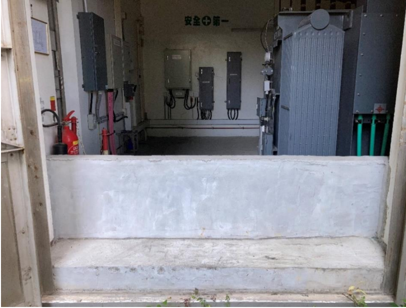
Flood walls are erected at existing distribution substations.
