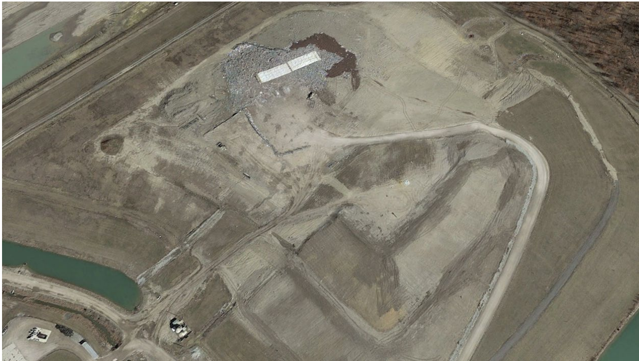
Figure 1. Working face area at an Ohio landfill using a tarp for daily cover.
