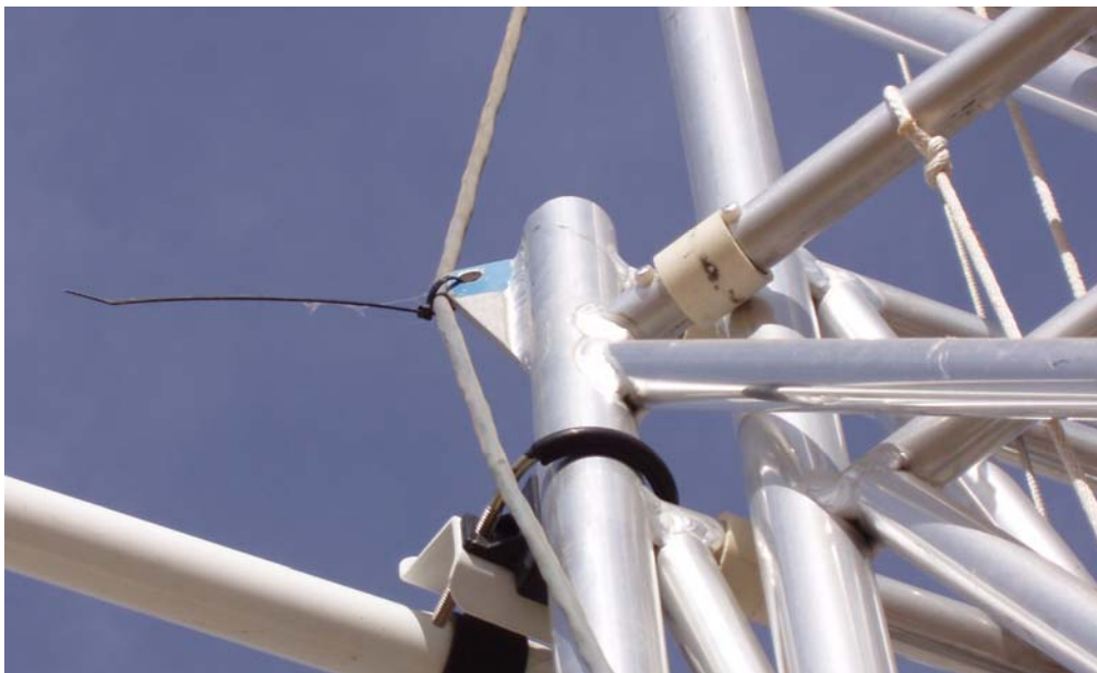
Figure 1.15 Wiring on a Crank-Down Tower
