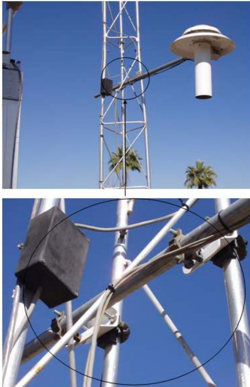
Figure 1.14 Temperature Cable Installation and Expanded/Close-Up Views
