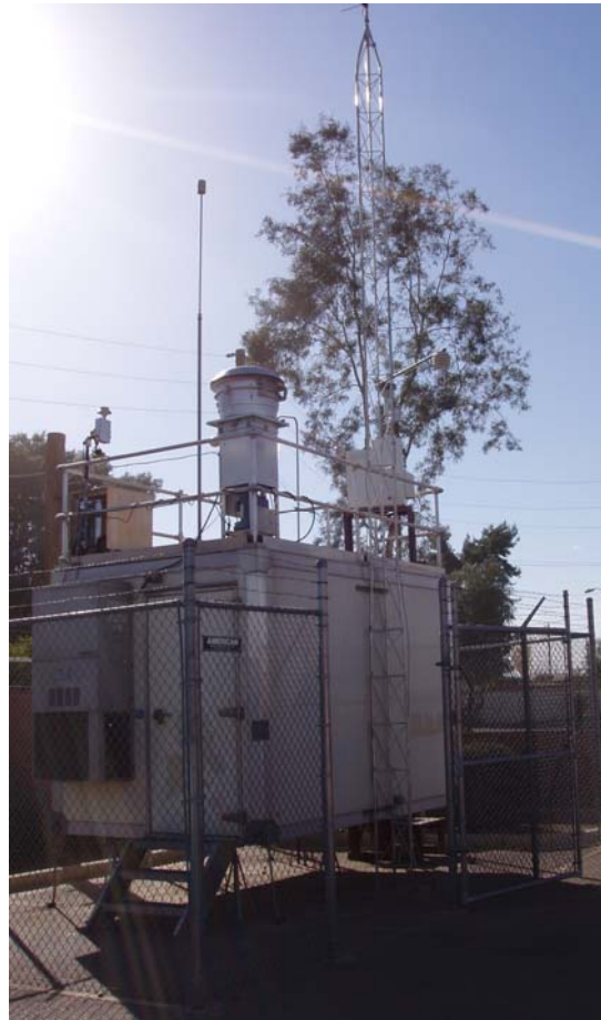
Figure 1.16 Example of a Tower Location
