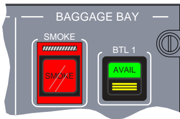
BAGGAGE BAY CONTROL-PANEL
