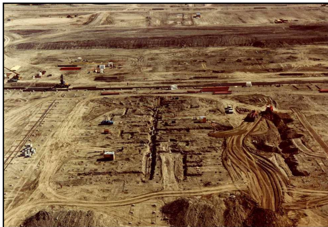
Figure 2-8 Example of Initial Excavation of a Refinery
