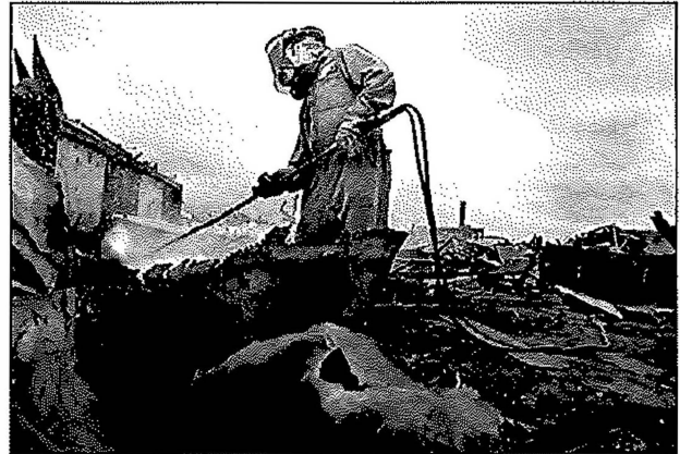
Worker torch-cutting scrap metal from vessel.
