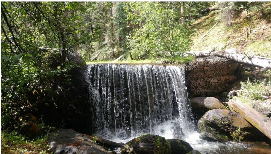
Protective gabion barrier on Paradise Creek, Arizona.
