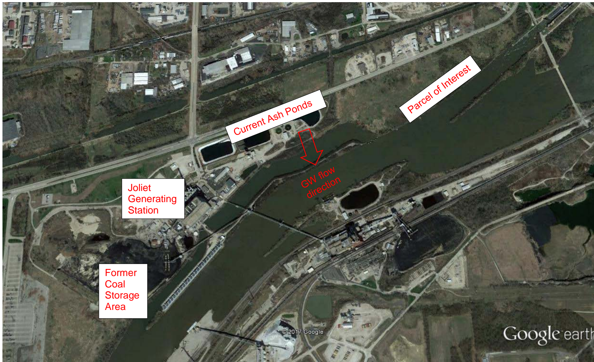
Figure N-7: Current Joliet Generating Station Facilities
