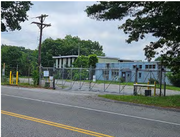
Eames Street - Olin Corporation Property 109 Eames St. (aka 51 Eames St.) Wilmington, Massachusetts
