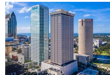
Park Tower Tampa, FL Renovated tower within heart of CBD
