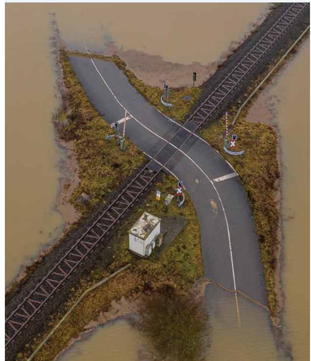
Flooding can disrupt critical transportation nodes, paralyzing transportation systems. Credit: Shutterstock
