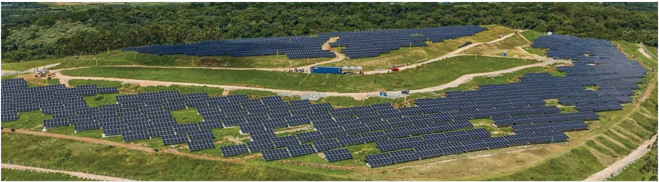
The C40 Finance Facility supported development of a solar plant on a deactivated landfill in Curitiba, Brazil. Credit: USAID
