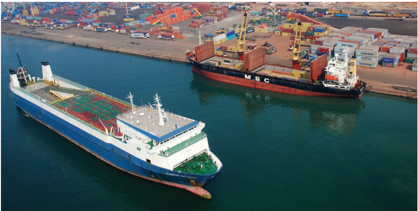
MCC's investments in Benin's Port of Cotonou attracted over $200 million in private financing, helping triple the port's capacity. Credit: MCC
