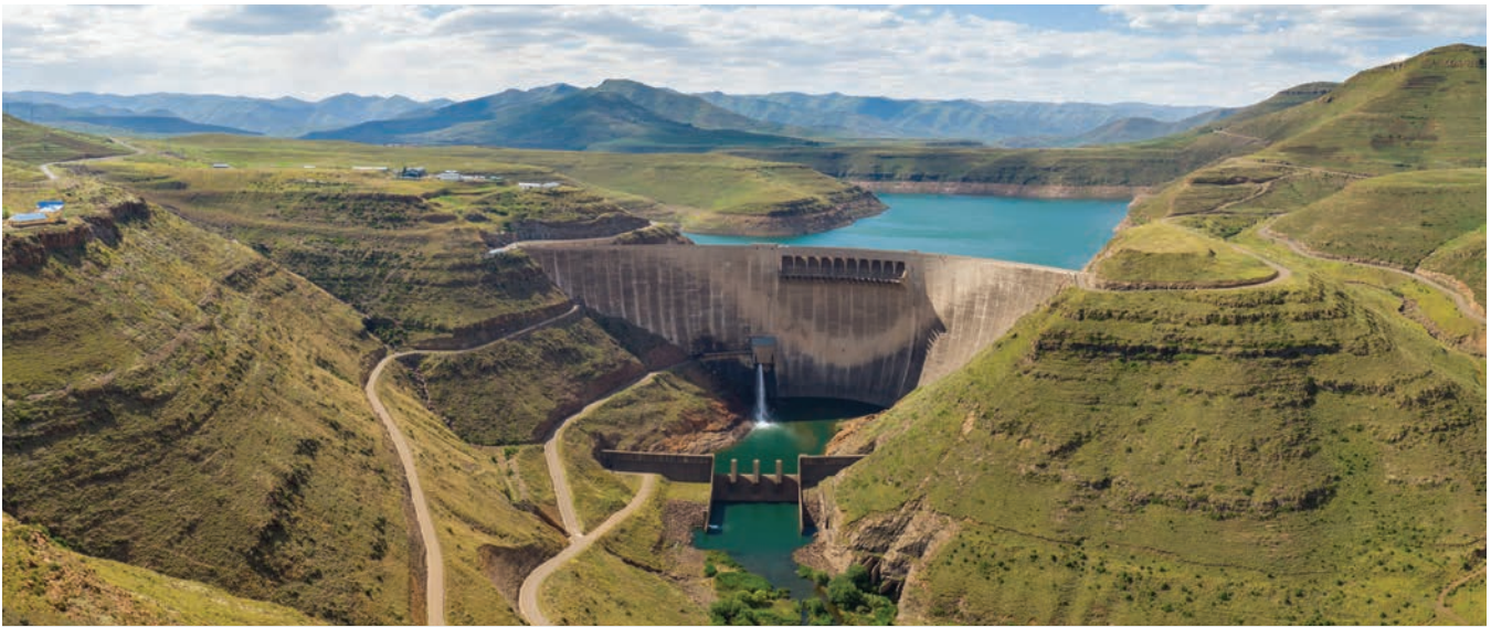
Dams exemplify how natural systems like rivers interact with built infrastructure systems such as energy generation. Credit: Shutterstock
