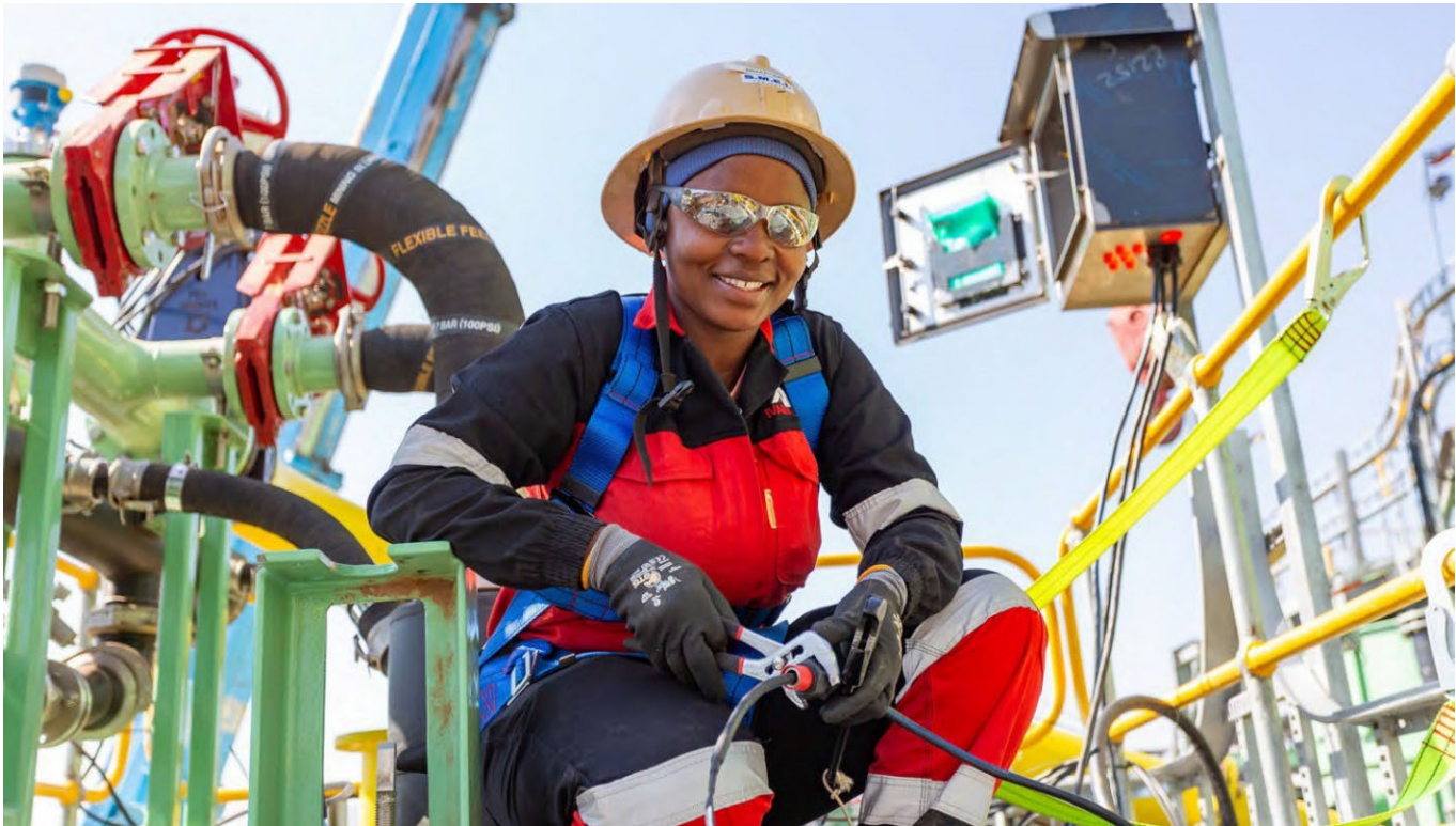
Photo: Electrician, Mapontsho Ngobeni, conducts testing at the Platreef Phase 1 concentrator
