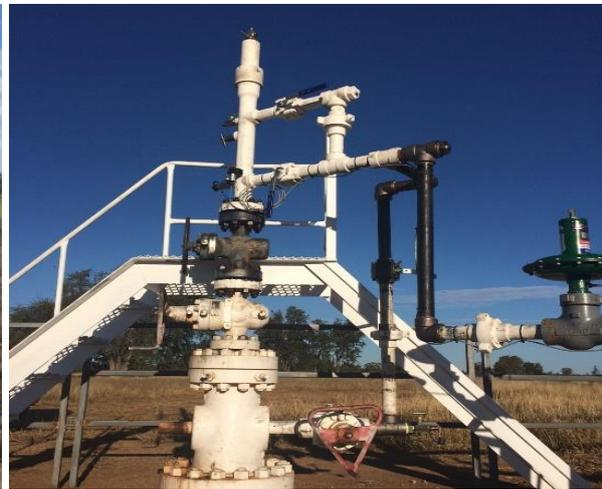
Fig 4: Plunger Lift Installation (June 2021)
