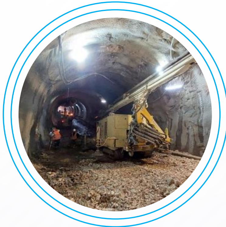
The main entrance tunnel
