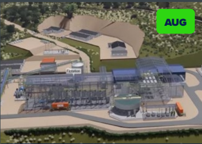
Epanko layout design completed for the 73,000tpa Graphite Processing Plant, Tailings Storage Facility and Water Storage Facility.
