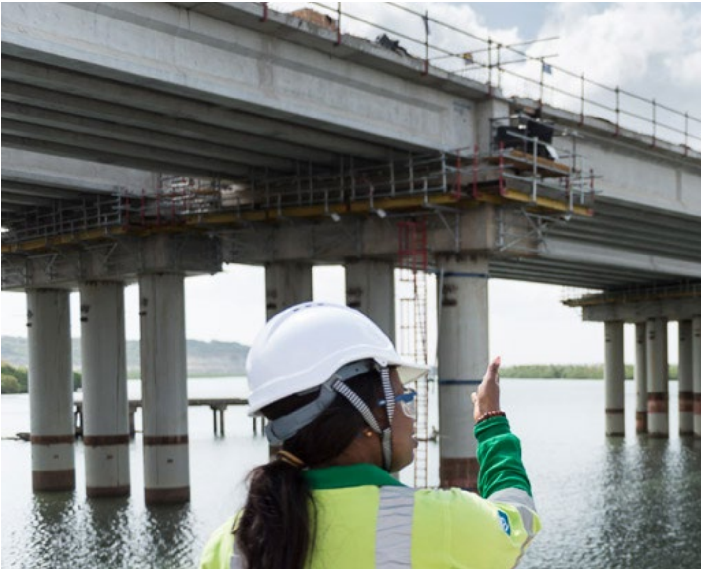
Bridging populations: The Dongo Kundu Bypass Highway was built using Power Crete, Power Plus and Duracem (for its durability attributes)
