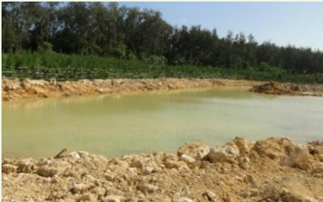
a.) New constructed wetlands in south quarry
