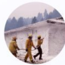
Firefighting Foam (AFFF)
