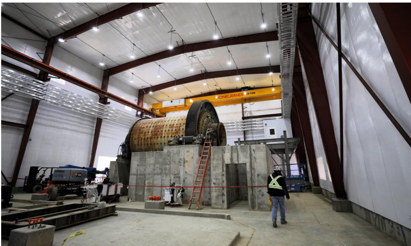
Figure 3 - Fully clad and weatherproofed mill building
