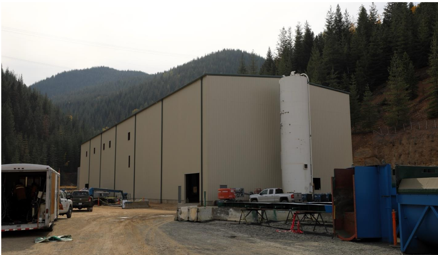
Figure 3 - Fully clad and weatherproofed mill building
