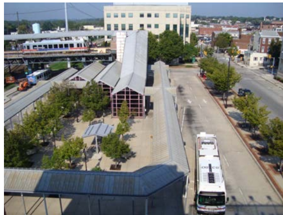
Sawtooth open bus bays at Norristown Transportation Center
