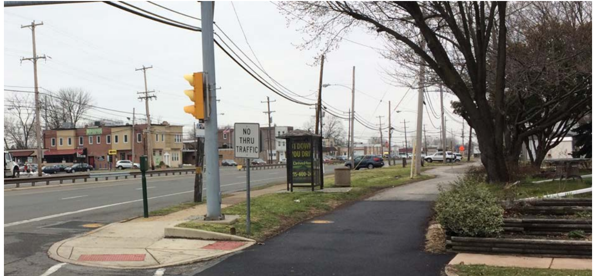
Pedestrian path and multiuse trail connecting to bus stop.
