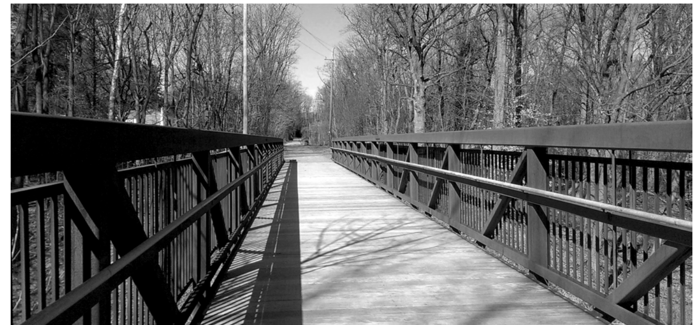
Description: Pennypack Trail on the inactive Newtown Branch Source: SEPTA
