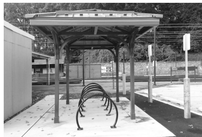
Description: Covered bicycle rack at Regional Rail Devon Station Source: SEPTA
