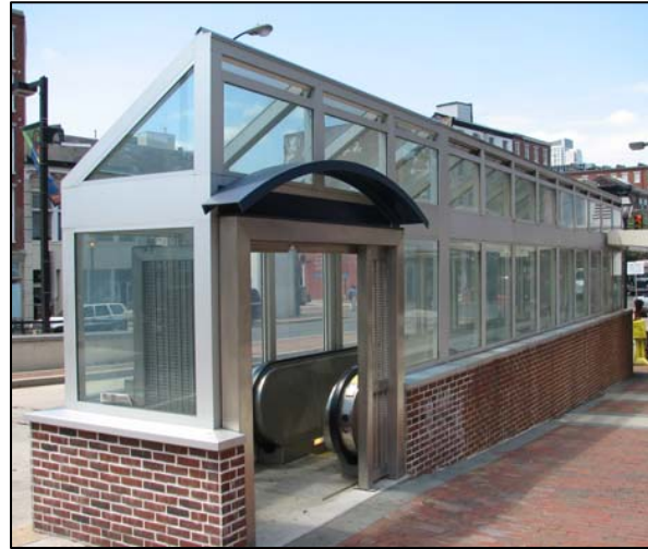
Market-Frankford Line 2 nd Street Station - New Escalator & Headhouse Extension
