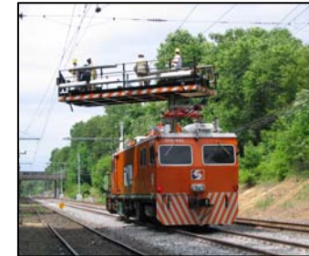
Regional Rail Catenary Replacement
