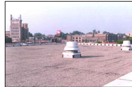
69 th Street Brake Shop and Motor Shop Roof Replacement
