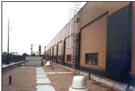
Wayne Junction Shop Roof Replacement and Siding Improvements
