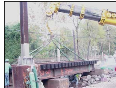
Bridge #5.74 Replacement R2 Warminster Line over Pennypack Creek
