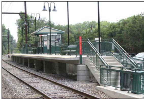
R5 Doylestown Line New Britain Station High-Level Platform
