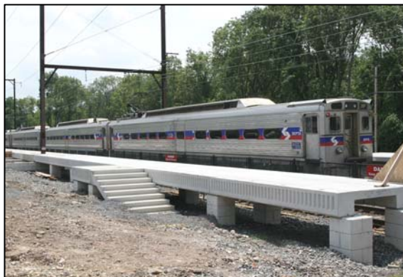
R5 Fort Washington Station Construction of High-Level Platforms
