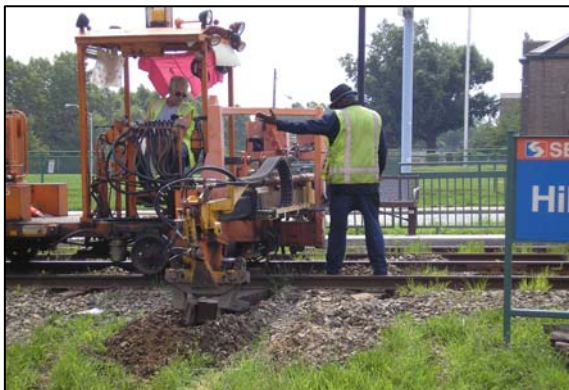
Media-Sharon Hill Line Installation of New Cross-ties
