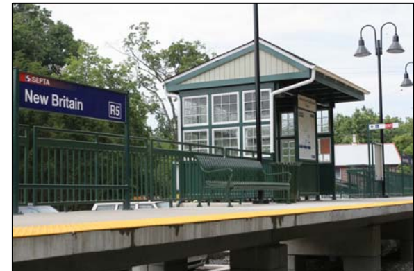
New Britain Station Construction
