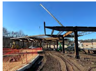
Construction of the new facility (Jan. 2024)
