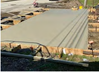
Overbrook Maintenance Facility Generator Installation
