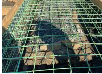
Overbrook Maintenance Facility 1
