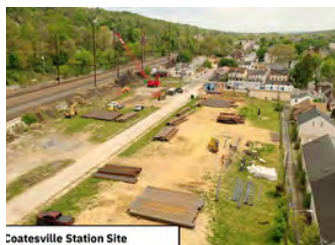
Coatesville Station Site Coatesville Station Site
