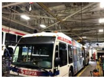
Maintenance Shop Equipment - Fall Arrest System
