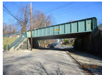
Image of MP 4.42 (Carpenter Lane).
