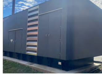
Overbrook Maintenance Facility Generator Installation
