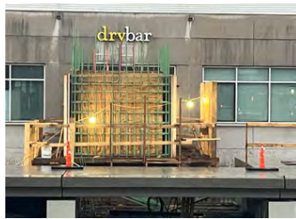
Construction on the future elevator wall.
