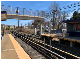
Existing conditions of the platform at Villanova Station on the NHSL.
