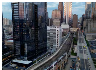
A SEPTA train traverses the Mainline Schuylkill Viaduct heading into Center City.
