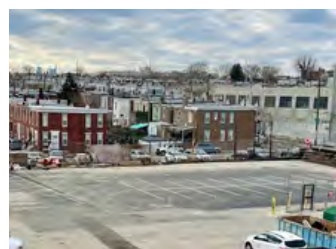
Completed paving and striping of the project.
