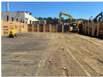
Excavation for the Wyoming Complex Stormwater Project.
