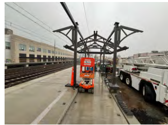
Construction on the canopy.
