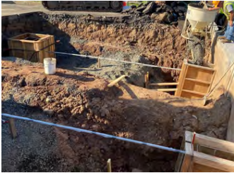
Warminster Platform Improvements
