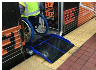
ADA Plates being utilized on a SEPTA station after installation.
