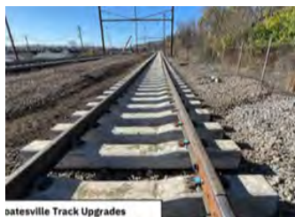
Coatesville Track Upgrades Track Upgrades at Coatesville
