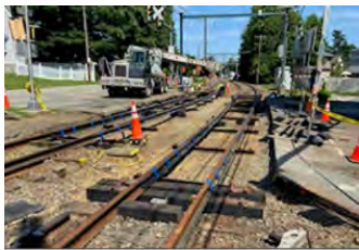
1/102 Positive Train Control and Right-of-Way Improvements Project picture
