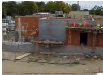
Construction on the Wayne Junction Static Frequency Converter building.
