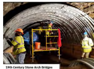
19th Century Stone Arch Bridges 19th Century Stone Arch Bridge
