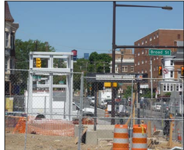
Allegheny Station Elevator Construction
