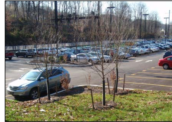
Exton Station Parking Expansion
