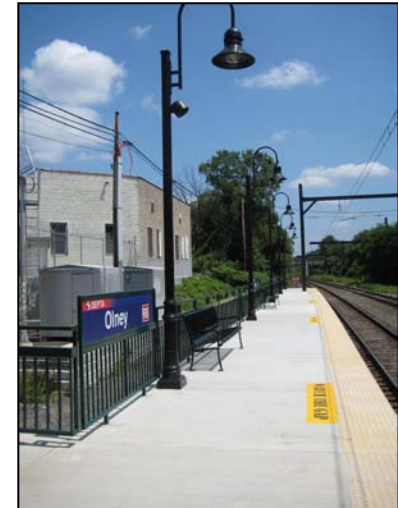
Completed Olney Station Fox Chase Line
