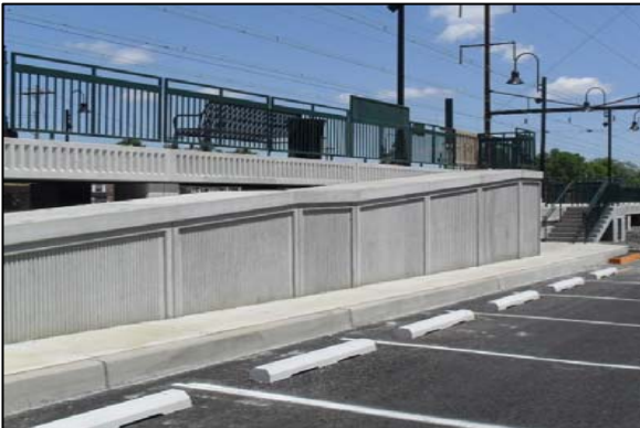
Croydon Station Renovations
