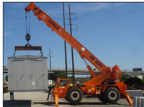
30-Ton Rough Terrain Crane
