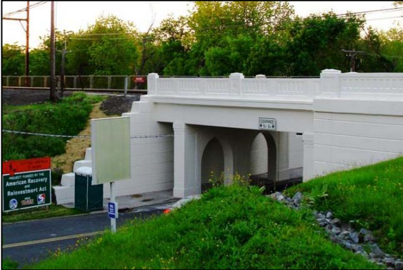
Lansdale – North Hills Bridge 13.04
