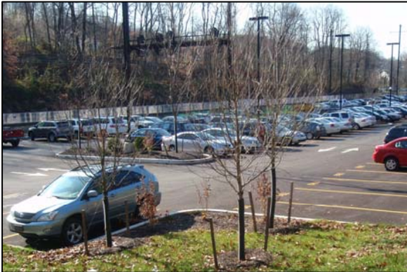
Exton Station Parking Expansion
