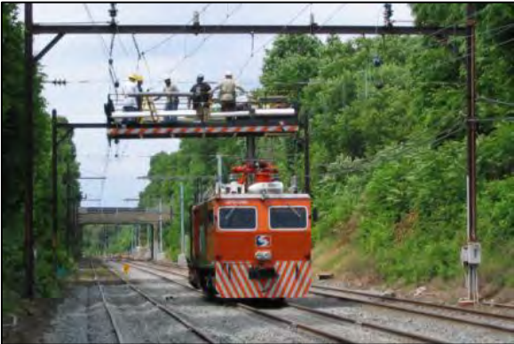
Catenary Renewal - Carmel
