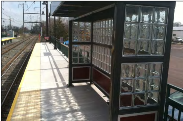
Primos Station Construction
