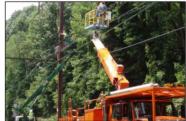
Catenary Work at Cane Interlocking
