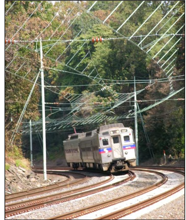
SEPTA Operation on Amtrak's Keystone Corridor
