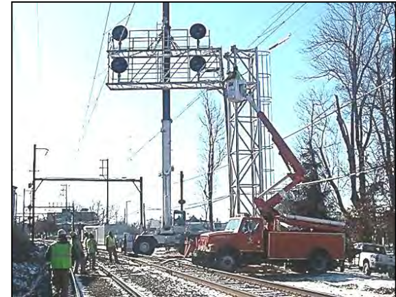
Signal System Modernization Warminster Line
