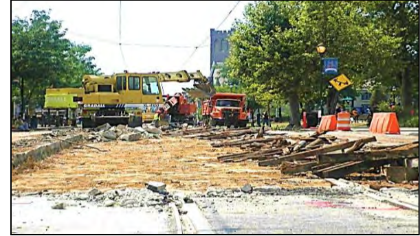
Route 34 Baltimore Avenue Track Renewal Project
