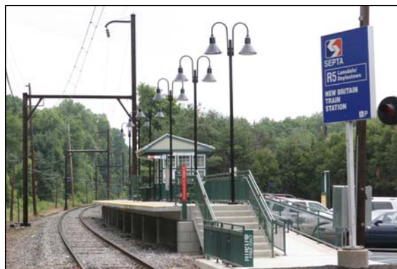
R5 New Britain Station High-Level Platform
