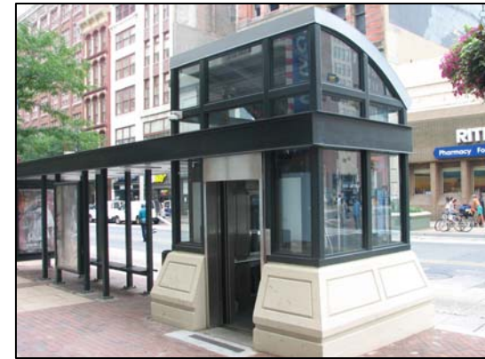
New Elevator at 8 th Street Station
