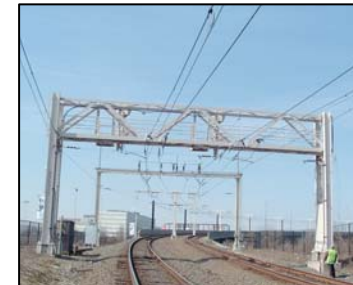
R1 Airport Line Catenary Replacement
