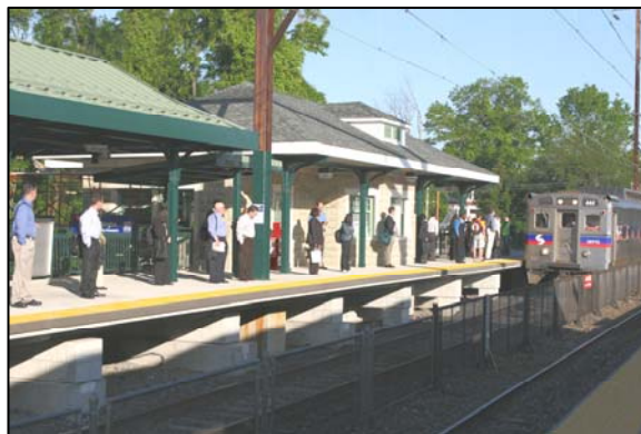
R5 Fort Washington Station Construction of High-Level Platforms
