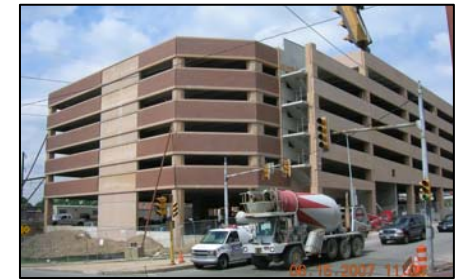
Norristown Transportation Center Parking Garage Construction
