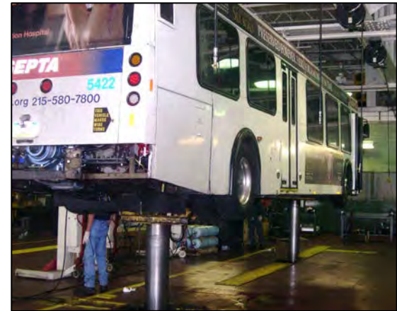
In-ground Bus Lifts at Berridge Shop
