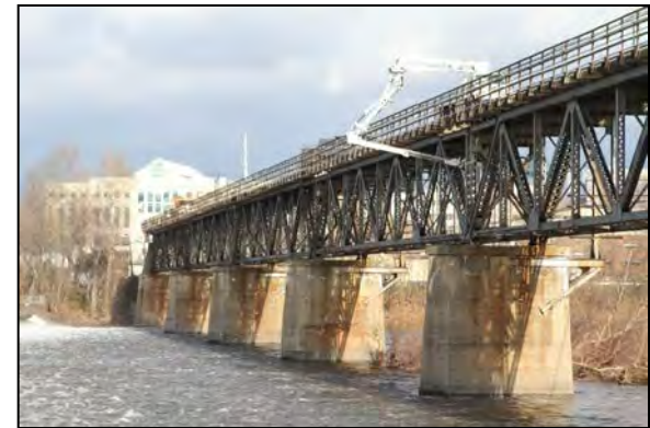
NHSL Bridgeport Viaduct
