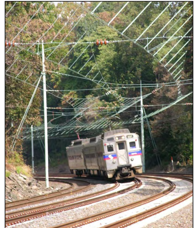
SEPTA Operation on Amtrak's Keystone Corridor
