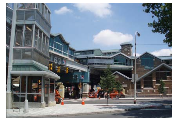
Market-Frankford Line 63 rd Street Station
