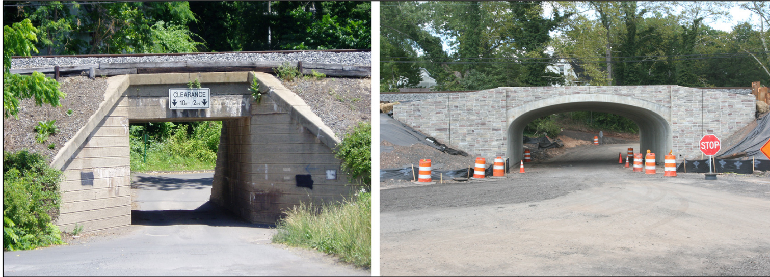
Lansdale Doylestown Line (R5) Bridge 8.53 at Delaware Valley College (Before & After)
