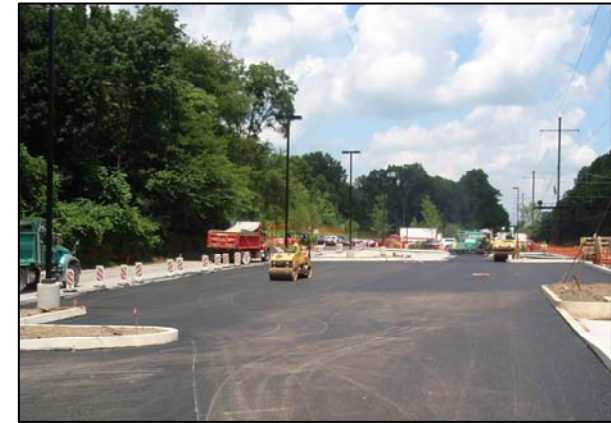
Exton Station Parking Expansion
