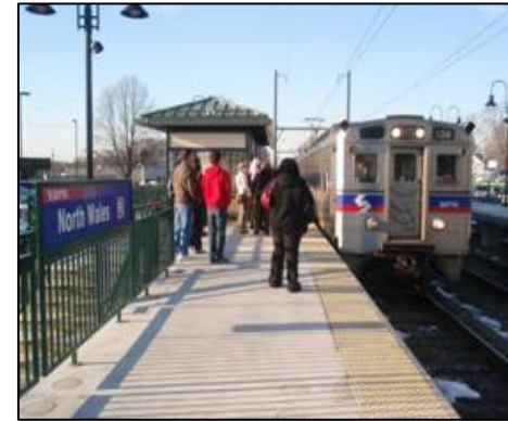
R5 North Wales Station
